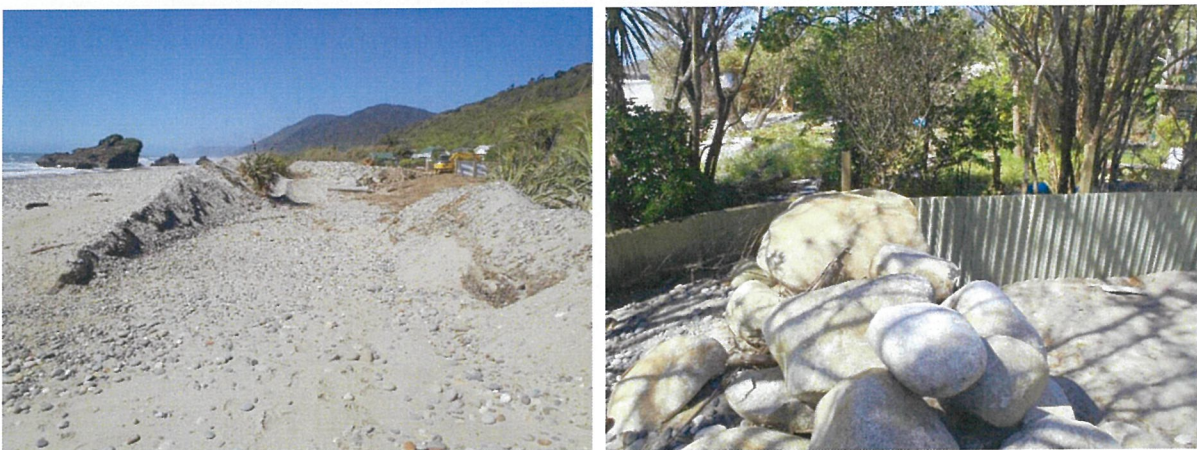
Figure 2 New ad-hoc defence along the beachfront (Left, 7 Main Road, Hector) and existing hard defences in reasonable condition (Right, Granity School). [Source: M Allis 22-11-2016].
