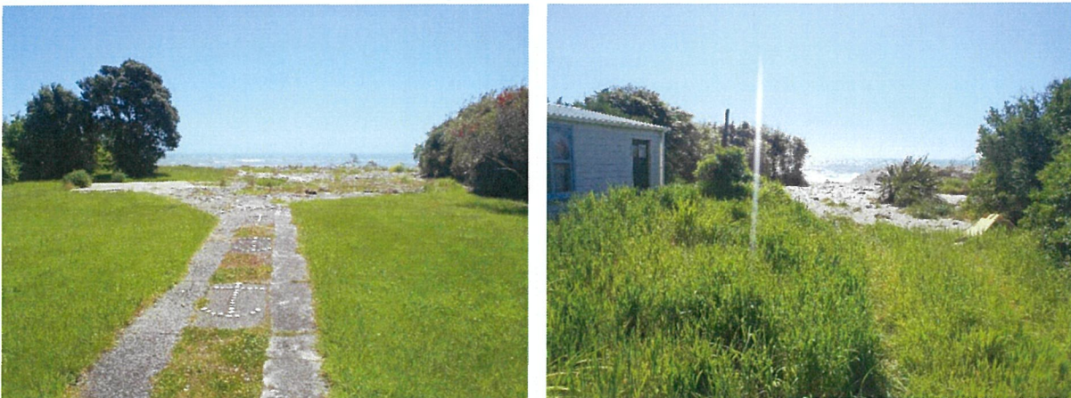
Figure 1 Recently deserted property (Left, 23 Main Rd Hector) and overwash evidence into private property (Right, 151 Torea St, Granity). [Source: M Allis 22-11-2016]
