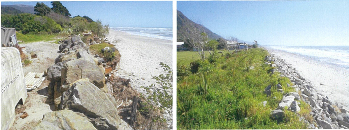
Figure 2 New ad-hoc defence along the beachfront (Left, 7 Main Road, Hector) and existing hard defences in reasonable condition (Right, Granity School). [Source: M Allis 22-11-2016].
